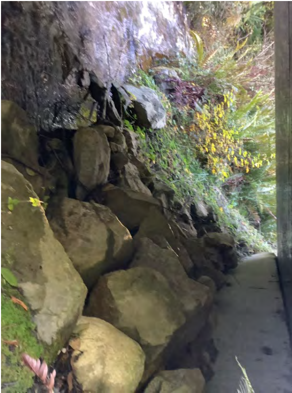
Right Bank Abutment when facing downstream
