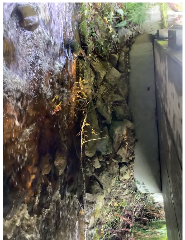
Left Bank Abutment when facing downstream
